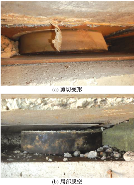
图 1 吕梁环城高速郭家沟 1 号大桥支座病害 Fig.1 The pad bearing disease of the No. 1 bridge of the Guo jia gou
