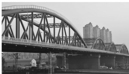
图 1 在役曲弦下承式钢管混凝土桁梁桥 Fig. 1 The working curved chord concrete filled steel tubular truss bridge
